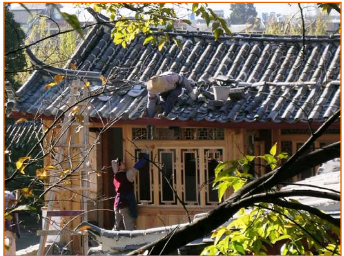
Lijiang, Yunnan Province, 2010 – Restoration of an ancient roof
